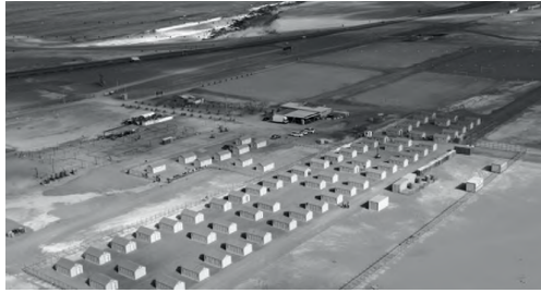
Photograph 8. Paper Log House, Kobe, Japan, 1995. Image by Takanobu Sakuma
