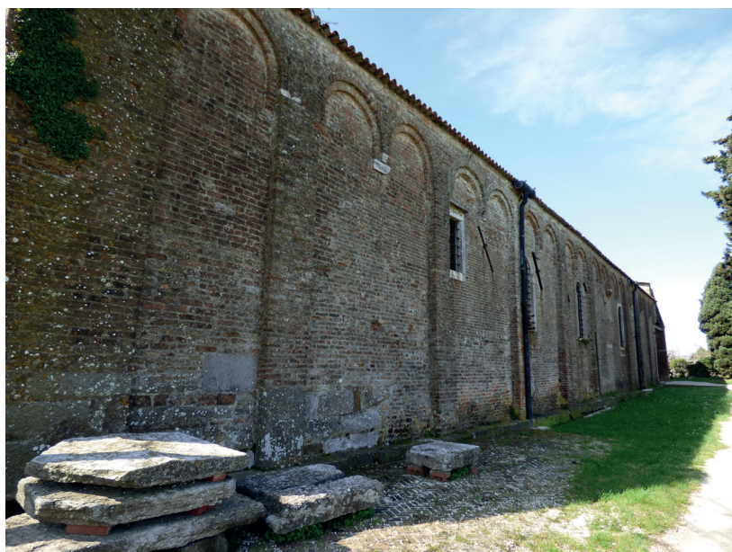
Fig. 17. A view on the external walls of the northern aisle of the Basilica di Santa Maria Assunta on Torcello (photo A. Krauze-Kołodziej)
