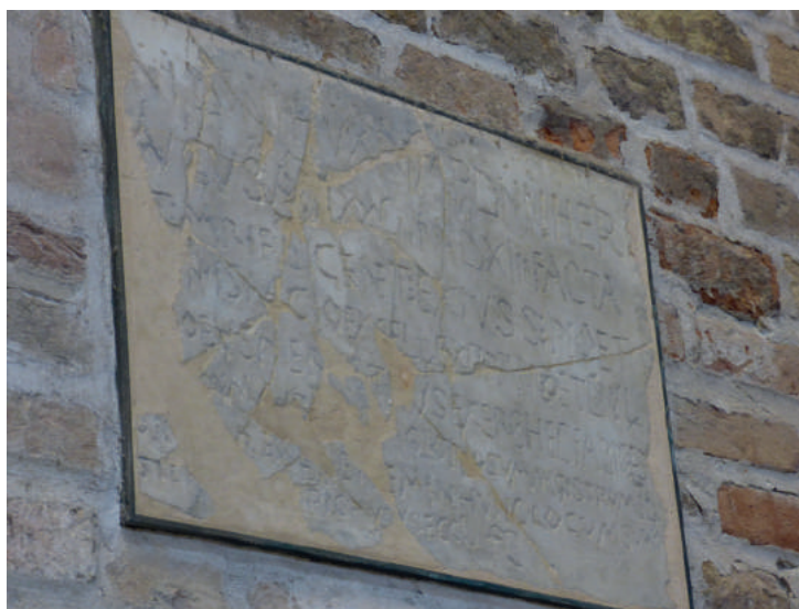
Fig. 28. The so-called foundation inscription on the left wall of the presbytery in the Basilica di Santa Maria Assunta on Torcello (photo A. Krauze-Kołodziej)
