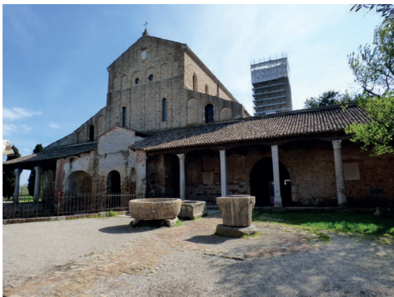
Fig. 2. The portico and the archeological remains of the baptistery in front of the Basilica di Santa Maria Assunta on the island of Torcello (photo A. Krauze-Kołodziej)
