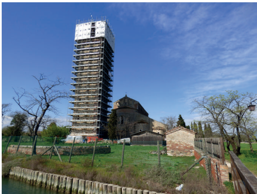
Fig. 10. The view on the bell tower, so-called St. Mark's Oratory, and the eastern part of the Basilica (photo A. Krauze-Kołodziej)
